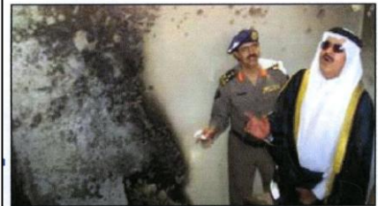
The Mecca city governor visited the fire-damaged school
